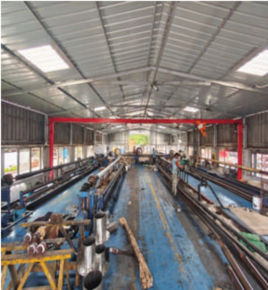
Hose Plant – Modification
