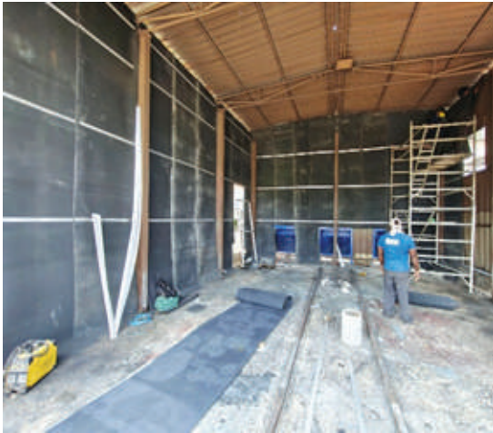
Renovation of Blasting Room
